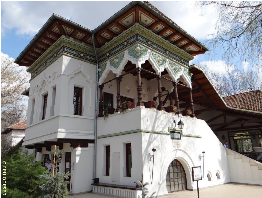
Casa Doina – Doina House, by famous architect Ion Mincu, built in 1892, is a famous restaurant in Bucharest.
